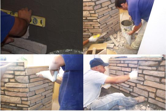
Fill in all joints between stones using a grout bag. After joints have become firm to the touch, use a blunt instrument to partially rake out the joint.
