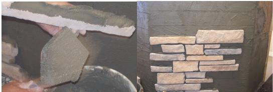
Apply the mortar to the back side of stone to be placed, press stone firmly to adhere the stone onto the surface. Using a level is very important on some types of stone.
