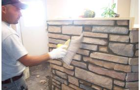
Finish smoothing and cleaning joints with a stiff brush. Using the same brush clean the face of the stone before the grout permanently hardens.
